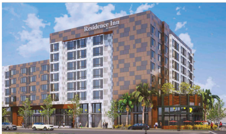
A.C. & RESIDENCE INN Fremont, California
