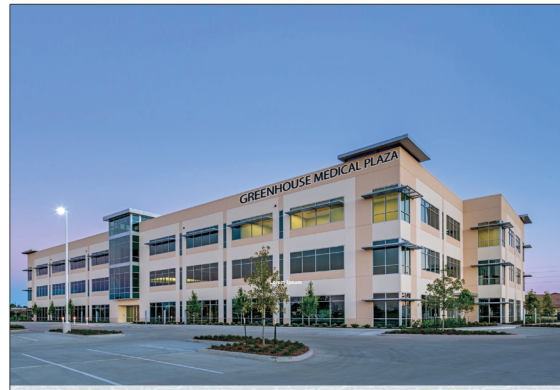
MRI GREENHOUSE Houston, Texas
