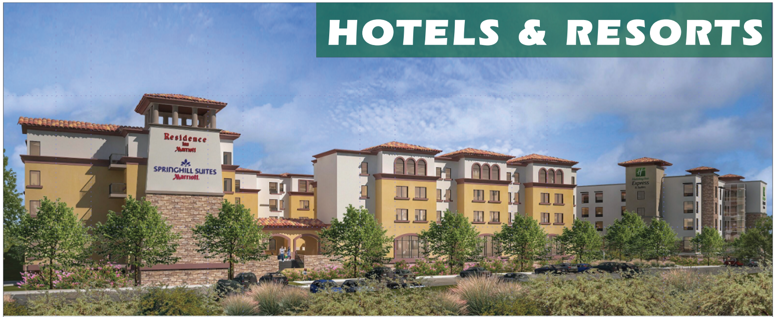
RESIDENCE INN, SPRINGHILL SUITE Santa Clarita, California
